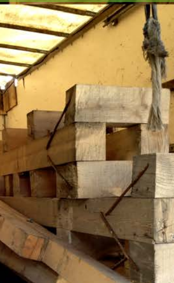
A truck of beams to be offloaded, sorted and stacked.
